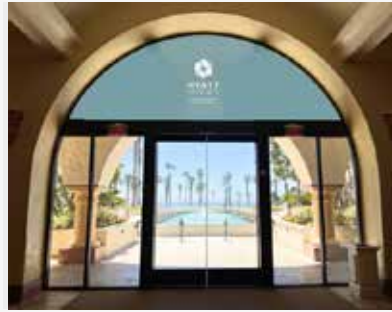
Main Lobby Courtyard Doors: Arch
